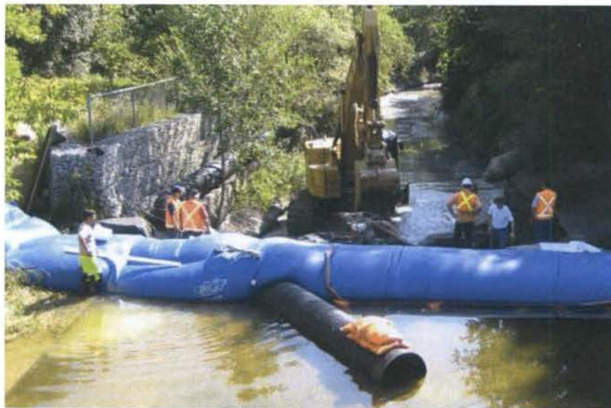
Figure 3. Photograph of a similar, water-inflated diversion dam courtesy of Hydrological Solutions, Inc.
